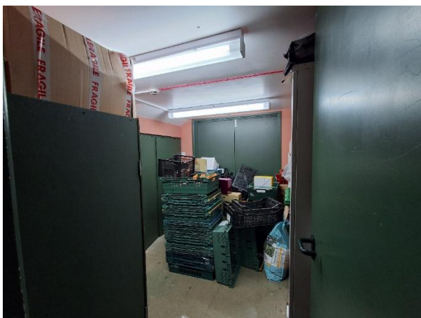
Store below small mezzanine
