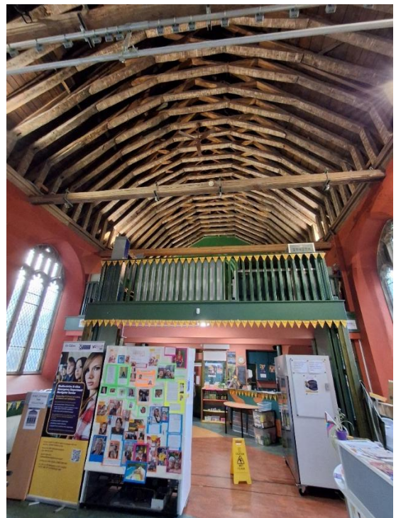
Nave, looking West, showing large mezzanine above shop area
